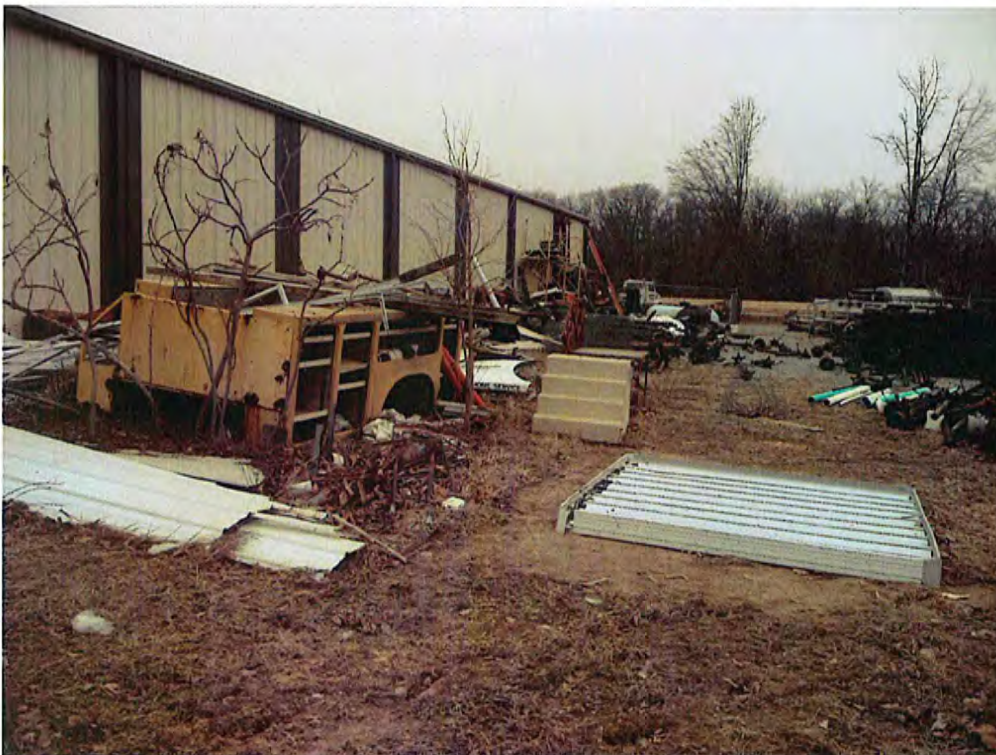
Date: 01/31/2014 Time: 2:52 p.m. Direction: N Photo by: M. Stevenson Exposure #: 020 Comments: yard on east side of building, metals, truck frame, pvc piping, miscellaneous waste.
