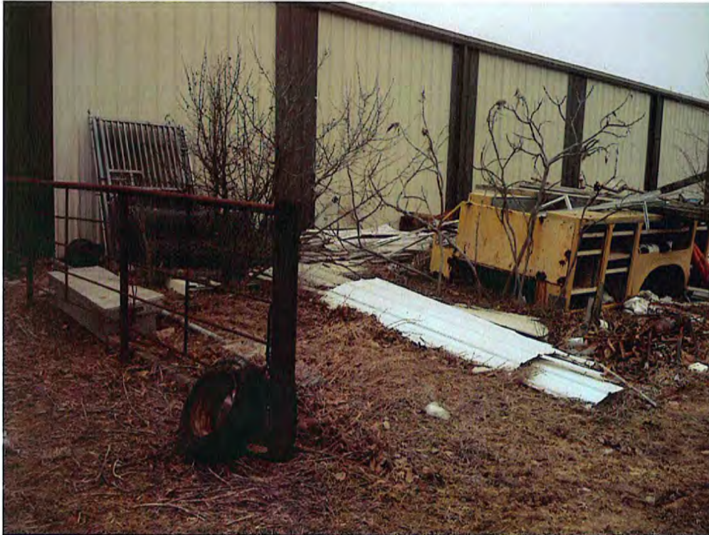
Date: 01/31/2014 Time: 2:52 p.m. Direction: NW Photo by: M. Stevenson Exposure #: 019 Comments: tire, metal siding-roofing, metal frame from truck, miscellaneous waste.
