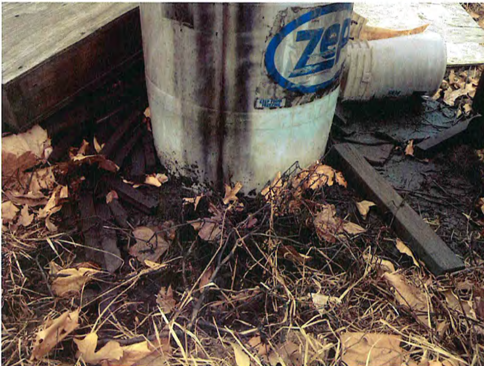
Date: 01/31/2014 Time: 2:53 p.m. Direction: SW Photo by: M. Stevenson Exposure #: 026 Comments: overflow markings on drum, spillage of fluid on ground, fluid soaked rags, fluid soaked dimensional lumber.
